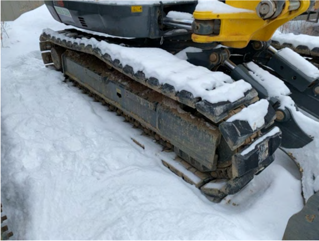
Right Track Condition / 02-15-2021
